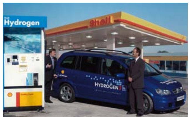
Shell hydrogen service station, Washington, DC
