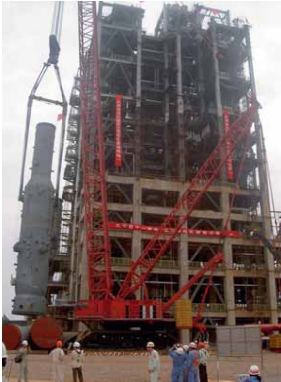
Figure 4. Shell Gasifier (2000 tpd) being installed at Yue Yang, China
